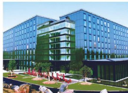
Residential apartment built in 3 days • Hubei
